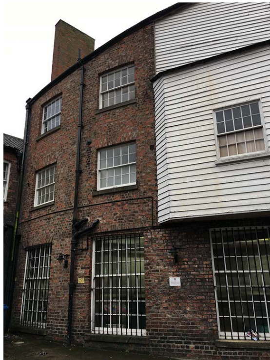
Figure 13 Rear (east) elevation of the De Grey Rooms, showing the large ground floor windows, and shuttered timber projection at first floor level.
