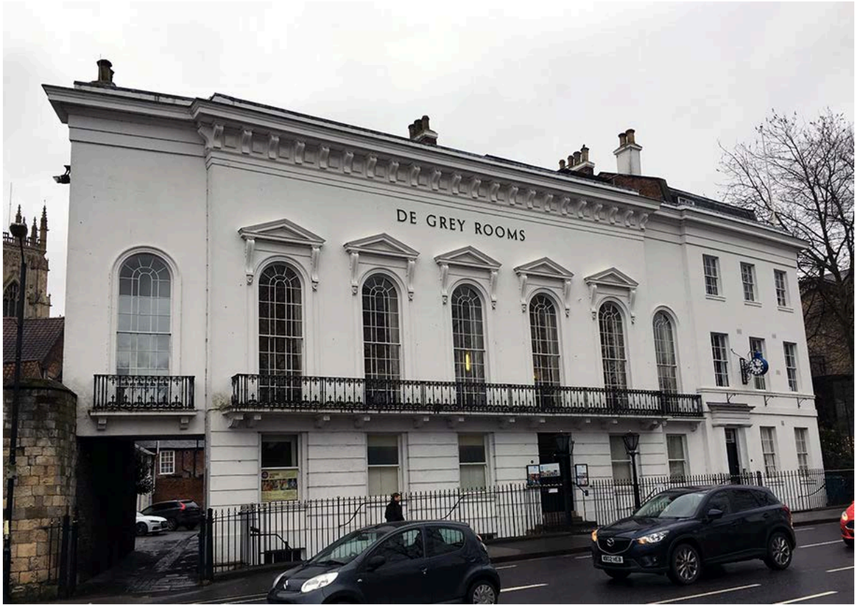
Figure 12 The principal (west) elevation of the De Grey Rooms with De Grey House on the right. Note the proximity to York Minster and the City Walls.
