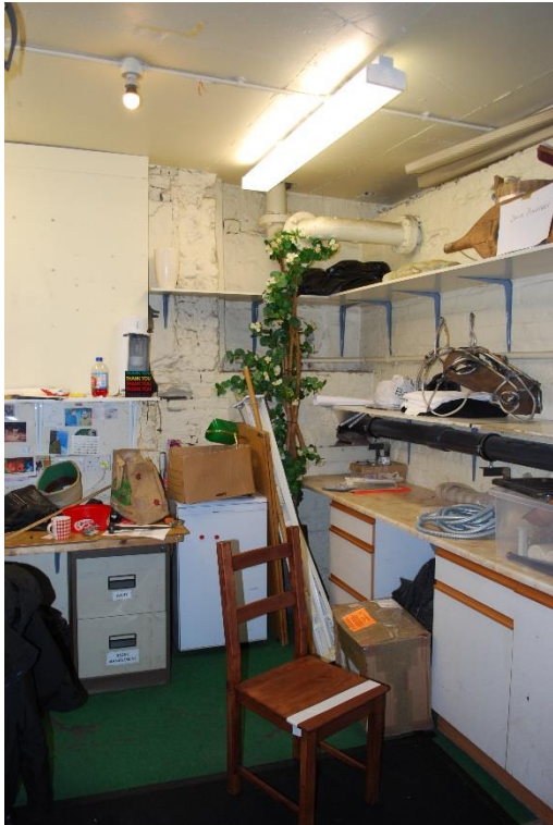
Blocked opening/window in rear office.
