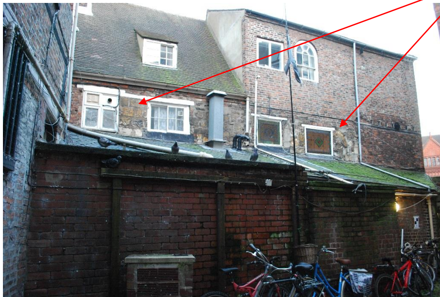
The former Manager's House, east elevation.
