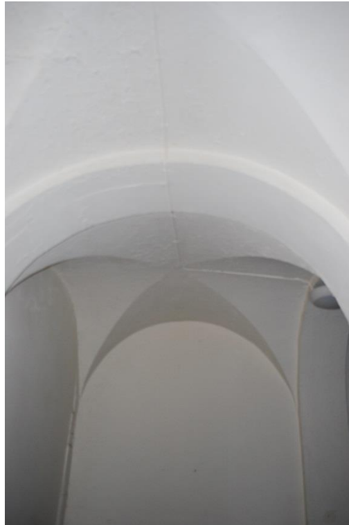
Groined vaulting on main stair.
