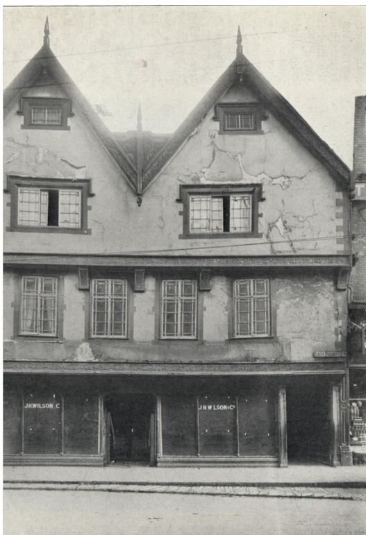
Figure 10 Mid C19 (1860s?) photograph of Herbert House, showing the painted quoins and window surrounds, as well as the C19 shop front, replacing the C17 shops visible in the earlier etchings. Note also the deterioration of the painted render (Reid 1926, 258).
