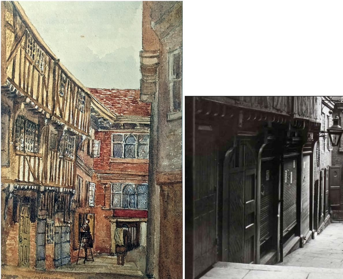
Figure 13 (left) Late C19 watercolour of Lady Peckett's Yard by Elizabeth Barstow (York Museums Trust); and (right) Detail from a 1902 photograph showing the ground floor of Building B, with herringbone brickwork, timber door, and roller shutters over the windows (© City of York Archives).
