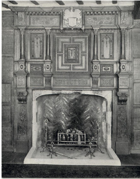
Figure 17 Restored fireplace in 1926 with herringbone brick lining to the firebox (Reid 1926, 257).
