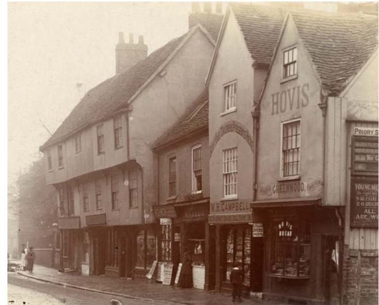
Fig. 5.3 Early C20th photo showing nos.85-89 fully rendered and with inserted sash windows and added signage over nos. 85 & 87 © York Explore
