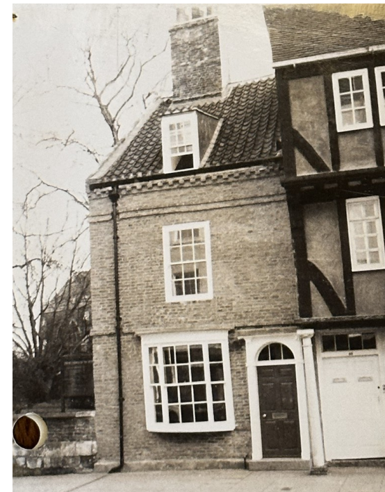
Fig. 5.27 Photograph from 1975 showing the fully restored no.83 Micklegate with the painted brickwork restored and the dormer window added.
