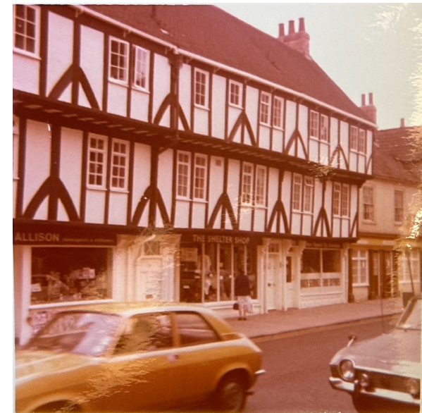
Fig. 5.22 Polaroid photograph of the fully restored nos.85-89 Micklegate.
