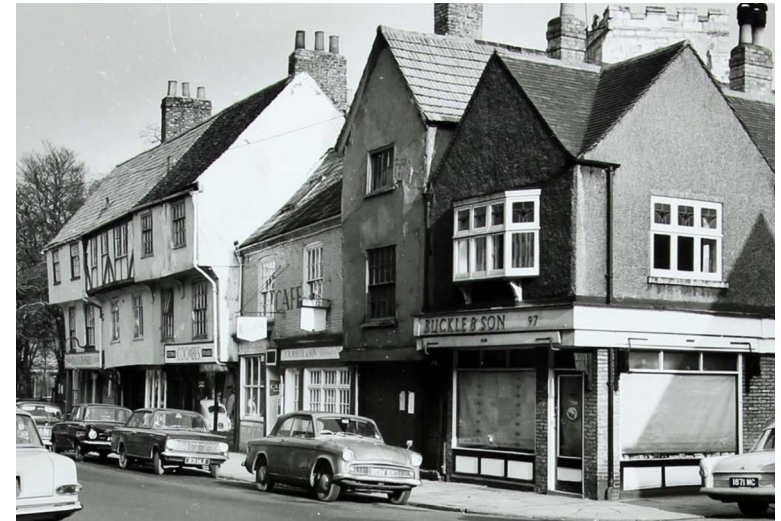
Fig. 5.17 Photograph from December 1965 showing that the render had been removed and the windows restored to the second floor of no.87 only © Historic England.
