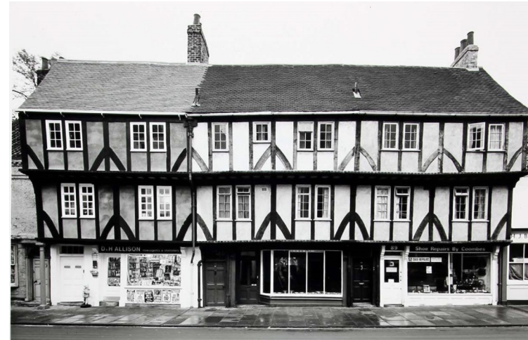
Fig. 5.12 Photograph of November 1969 showing the fully restored nos.85-89 Micklegate. No.83 has yet to be restored, and the new infill panels to no.85 are yet to be painted © Historic England.
