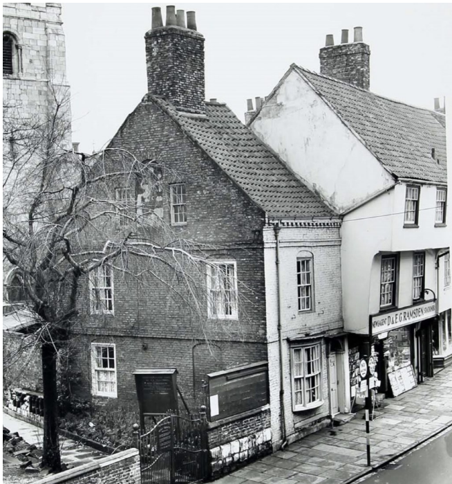
Fig. 5.26 December 1964 photograph showing no.83 prior to its restoration. Note the infilled ground floor window in the side elevation, and lack of rear extension © Historic England.
