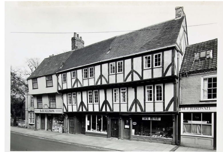
Fig. 5.18 Photograph of April 1967 showing the newly restored nos.87-89 Micklegate. Note no.85 has yet to be restored and retained its external render and sash window © Historic England.
