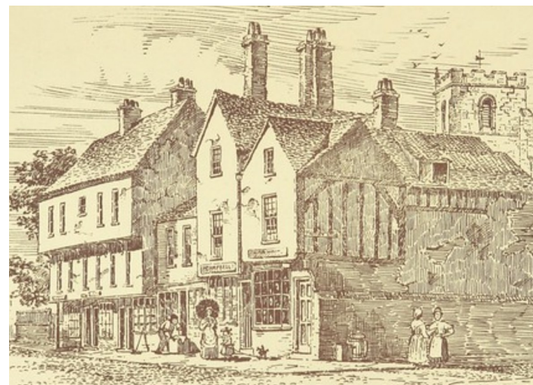
Fig. 5.15 Earliest known depiction of 85-89 Micklegate, showing it rendered with sash windows on the upper floors, with bowed shop front windows below. (Benson 1886).
