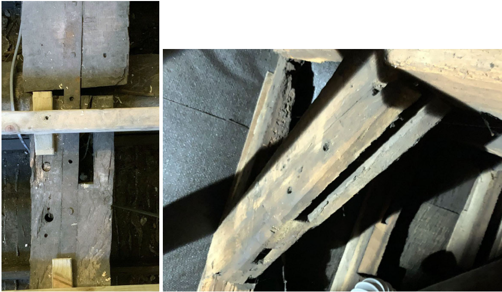
Fig. 4.2 Reused timbers as floor joists (left) and roof truss collar (right).
