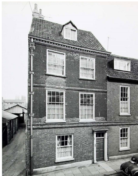
Fig. 4.12 Photograph of no.27 from June 1966 showing the rebuilt ground floor © RCHME
