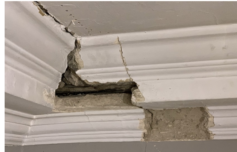
REPAIRS Example of plasterwork repairs to the North Anteroom cornice and ceiling in the Assembly Rooms. Damage has been raked out ready to hand run new lime hair plaster.
