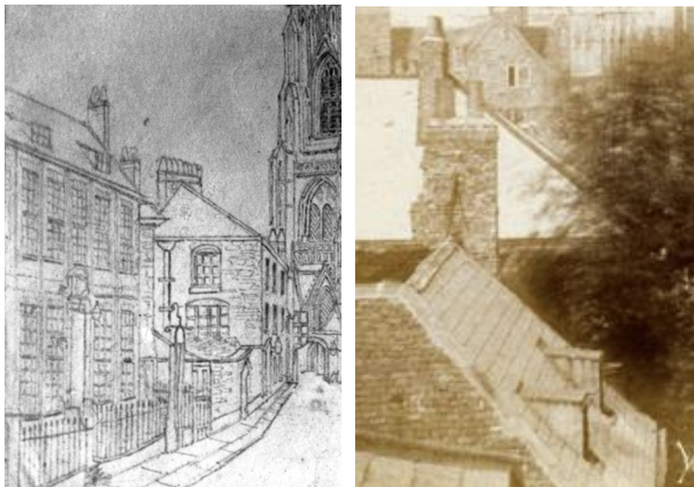
Figure 10 Left - early C19th etching of Lop Lane (now Duncombe Place) with the principal elevation of the site shown to the far left. Note the simple catslide dormers in the front roof slope, and the cast iron archway in the railings © YAYAS; Right - these plain dormer windows can be seen in this photo of c. 1859 across the rooftops of York © York Explore.
