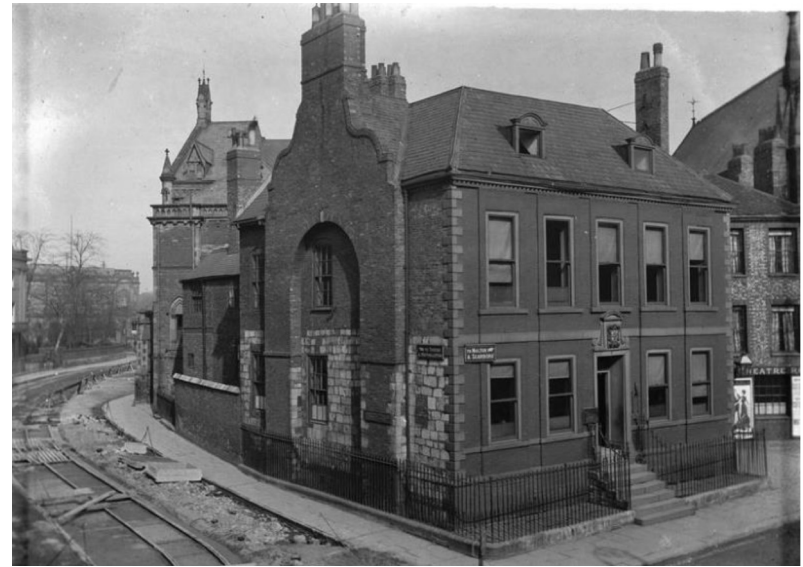
Figure 12 Photograph of c.1911 showing the site from the south. Note the replacement of the windows to the principal facade, but not the side elevation. Note also the cast iron railing along St Leonard's Terrace.
