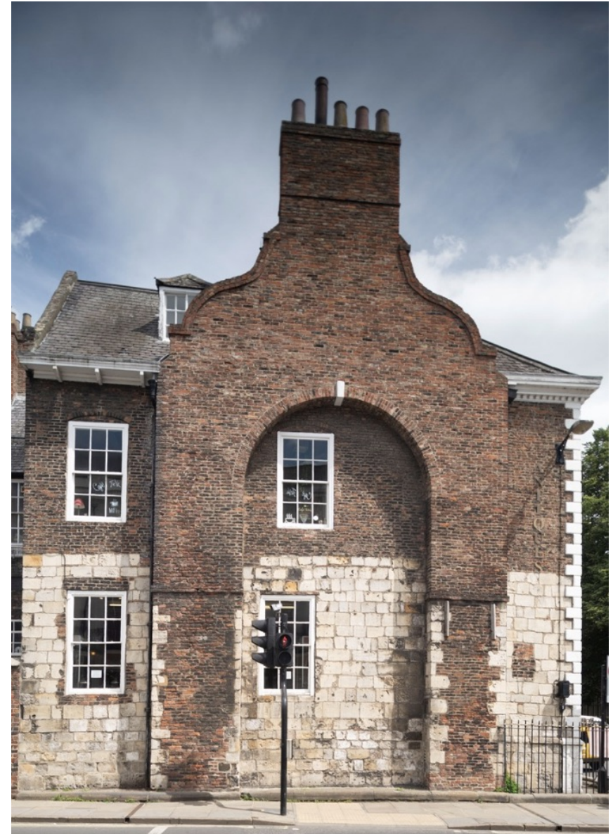
Figure 1 Part of the western elevation of the Red House ©YCT.
