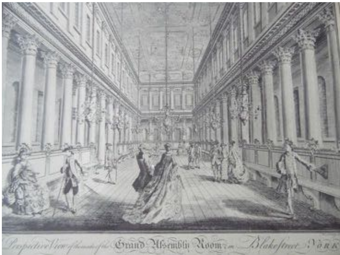
Fig. 2. 1760 Engraving by W. Lindley showing the Great Assembly Room with its plain ceiling. ?? Altered version of the Lindley's 1760 etching including a fanciful Rococo ceiling design.
