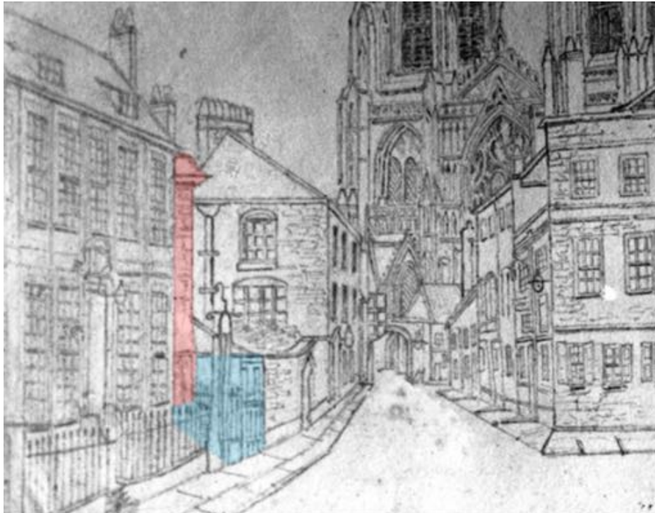
Fig. 2.7 Early c19th drawing of Little Blake Street prior to widening, appearing to show a wall and double gates (blue) in front of TWH (red) © YAYAS not for reproduction.
