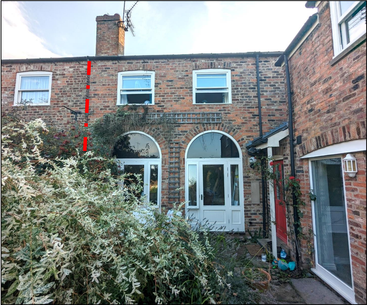
Figure 42. The more narrow, arching doorways of No. 2 The Mews in the center, with No. 1 to the left and No. 3 to the right. The red dashed line highlights the building break between Nos. 1 and 2. Summer 2023.
