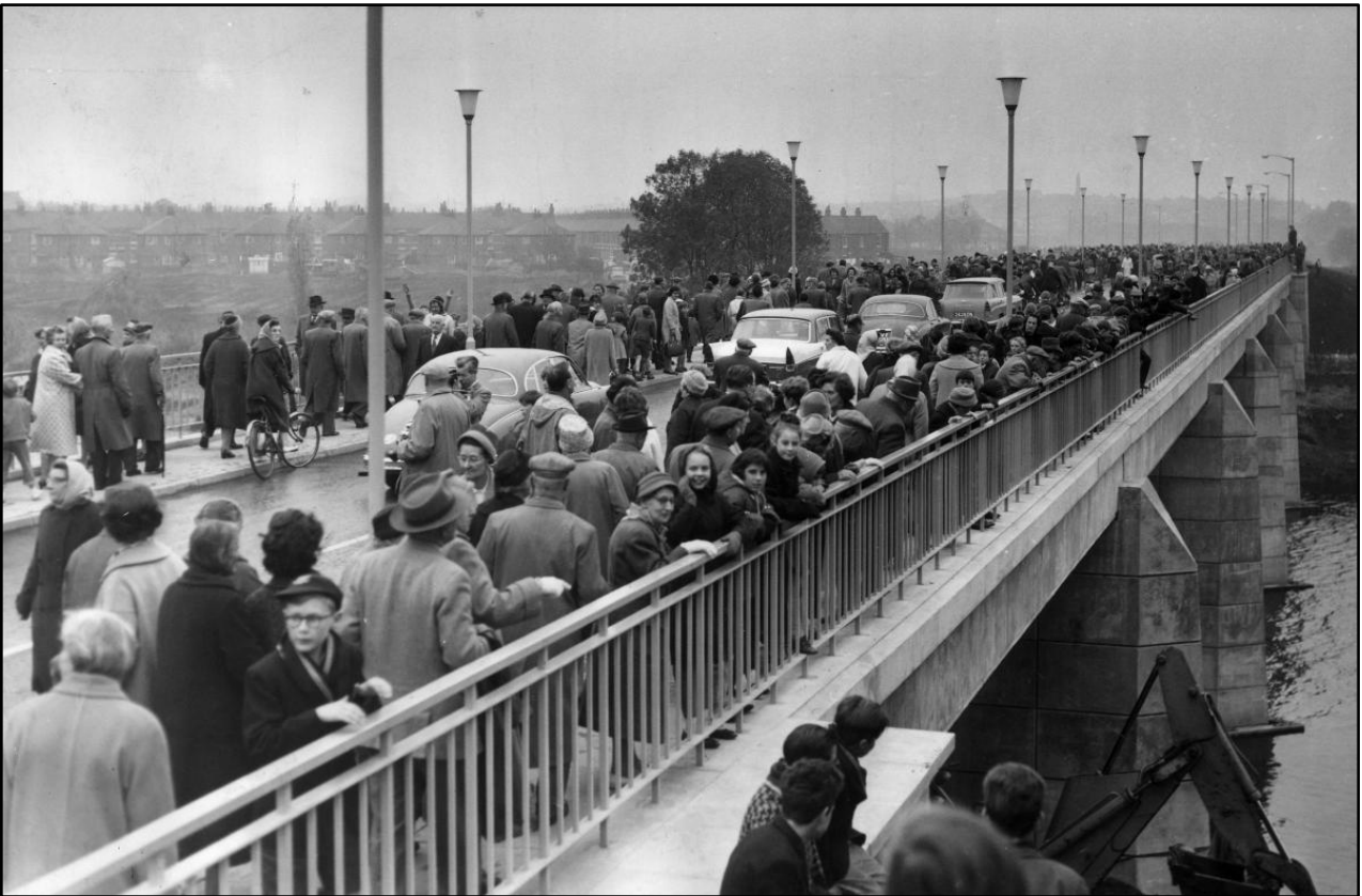
Figure 95. Clifton Bridge's opening in 1963 (Gordon 2023).
