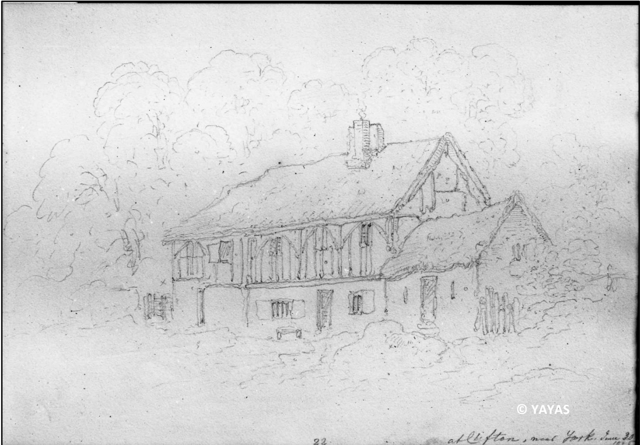
Figure 19. A timber-framed building in Clifton dated June 30 th 1825 by George Nicholson (YAYAS EV898).
