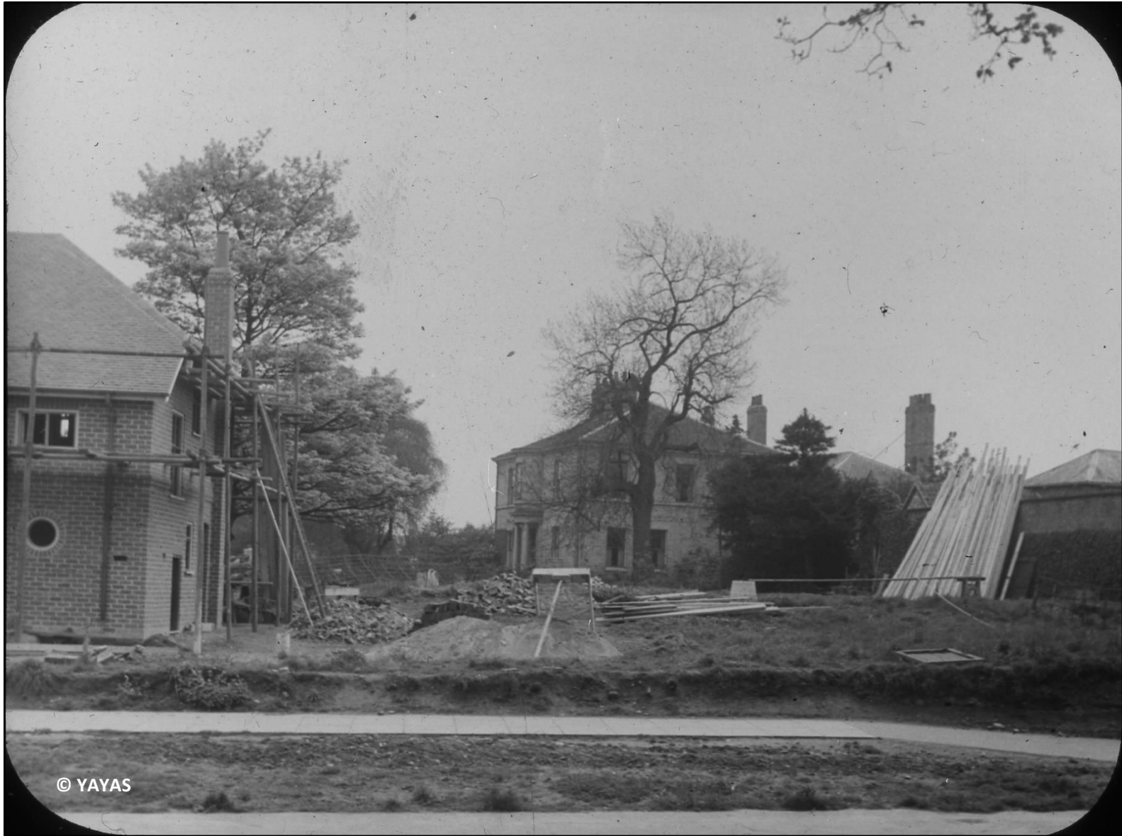
Figure 79. Clifton Croft from Water End, likely 1931-1932. No. 13 Water End can be seen under construction on the left-hand side of this photograph, while Clifton Croft is prominent in the center, with the hipped roof of the Stable Block (now No. 3 The Mews) on the right (YAYAS EV2817).
