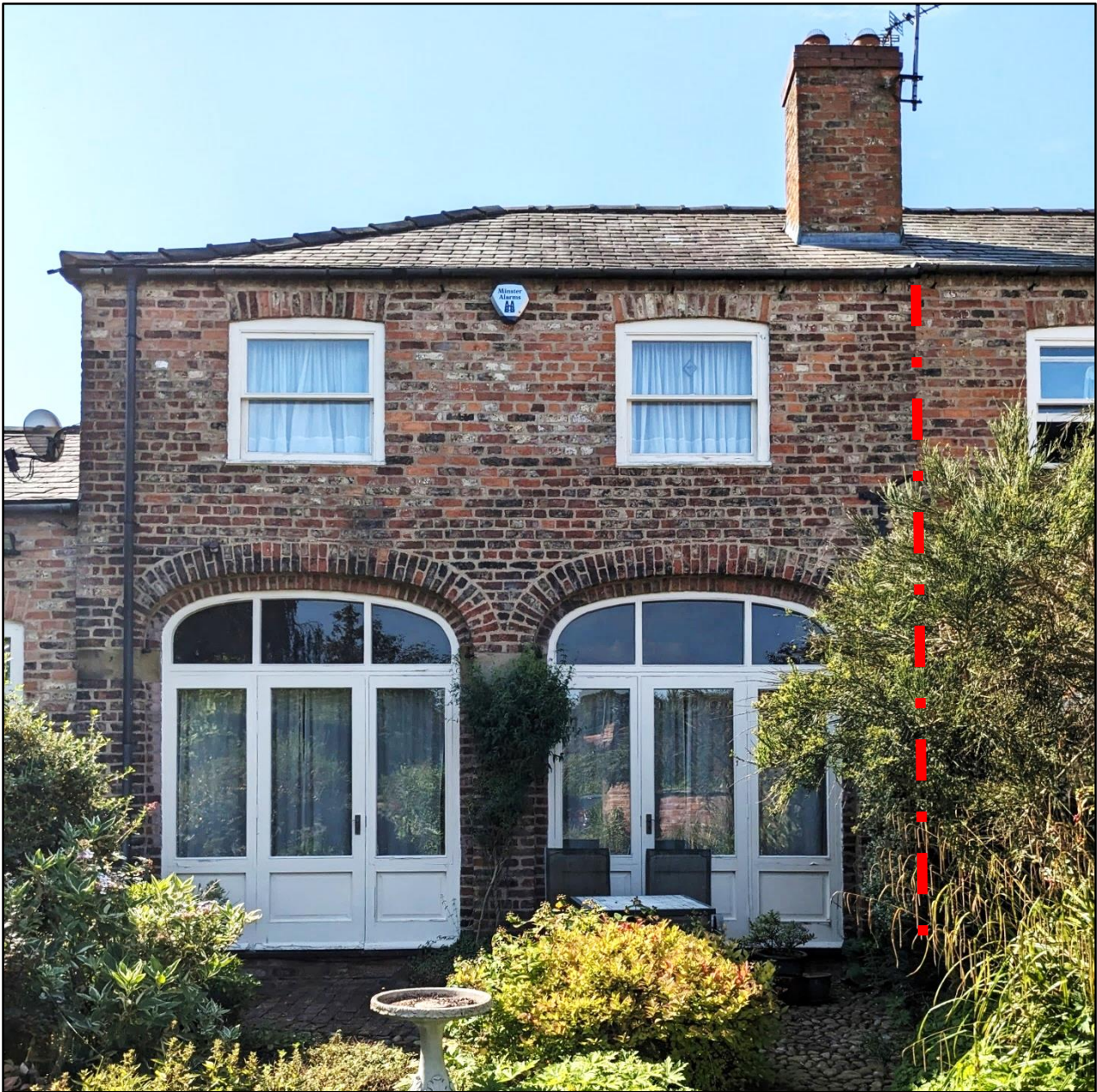
Figure 30. The higher doorways here mark the two-storey portion of No. 1 The Mews, likely originally a coach house. The building break between Nos. 1 and 2 is highlighted in red. Summer 2023.
