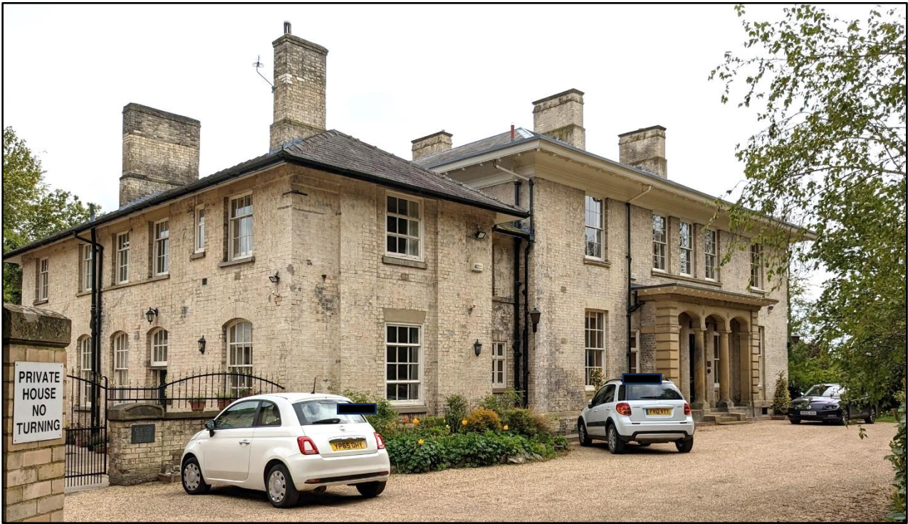
Figure 40. Clifton Holme, now St Hilda's Garth. The attached structure on the left is the service wing. Spring 2023.
