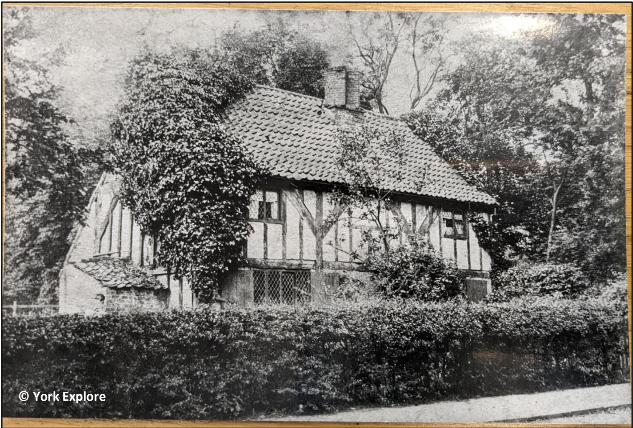
Figure 20. A timber-framed building in Clifton, photograph originally taken in 1898 (CYA HMU/P/9/7).
