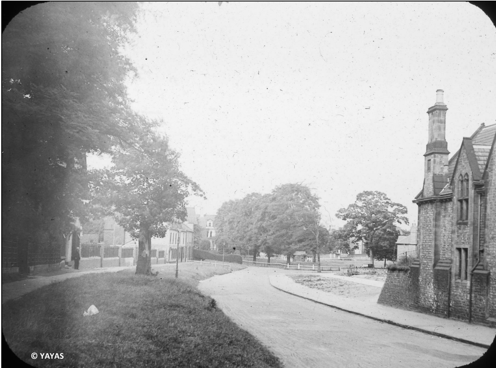
Figure 78. Water End, Clifton, likely 1931-1932. This photograph shows the Laborers' Cottage after land clearing and the demolition of the former boundary wall to the Clifton Croft complex. The pavement set back from the edge of road indicates the new line of Water End through the Laborers' Cottage (YAYAS EV2764).
