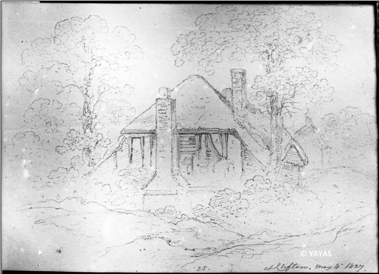
Figure 18. A timber-framed building in Clifton dated May 4 th 1827 by George Nicholson (YAYAS EV899).
