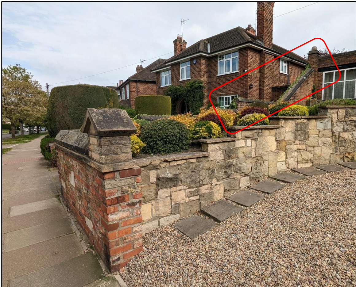
Figure 84. A portion of the brick wall that previously made up the northern boundary of the Laborers' Cottage and enclosure now part of No. 19 Water End. Summer 2023.
