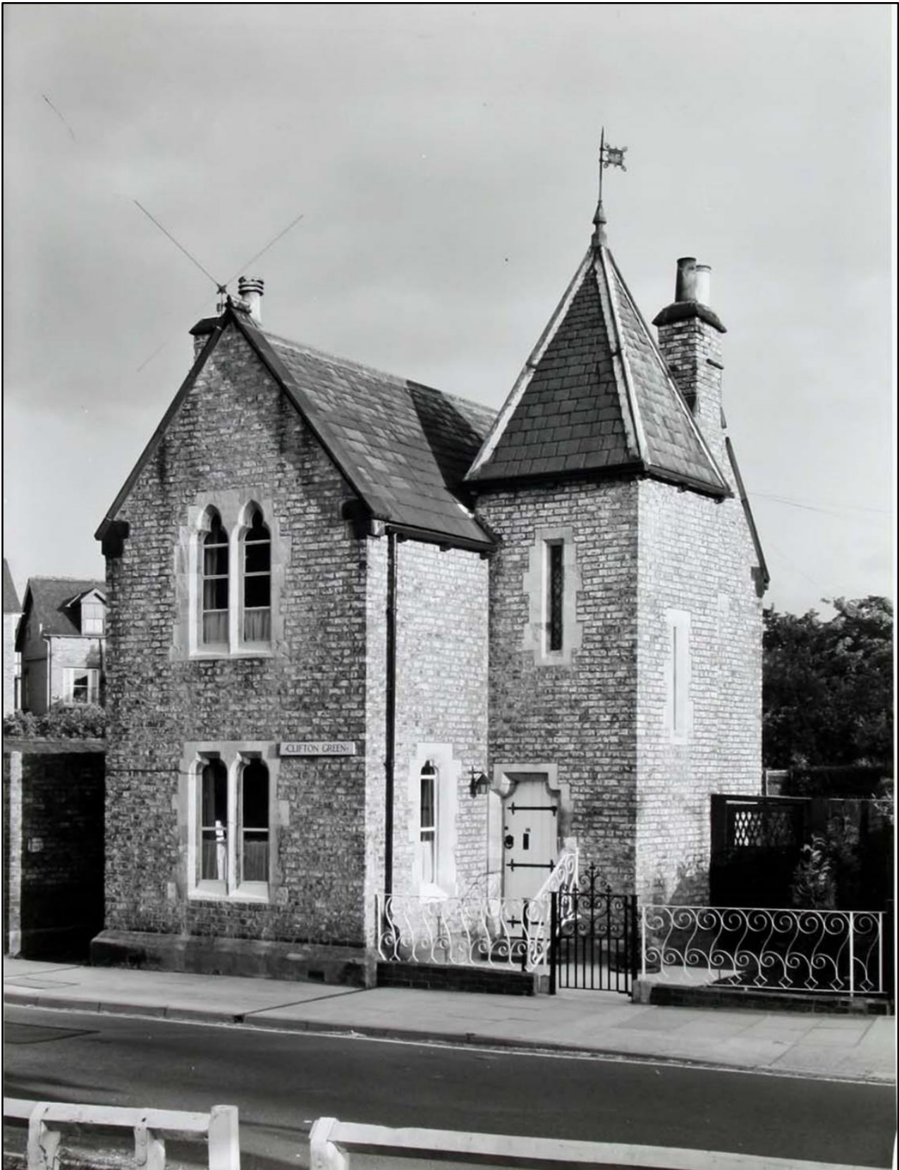
Figure 85. The Gardener's House, now No. 16 Clifton Green, in 1971 (Historic England 1971, 6527_151).
