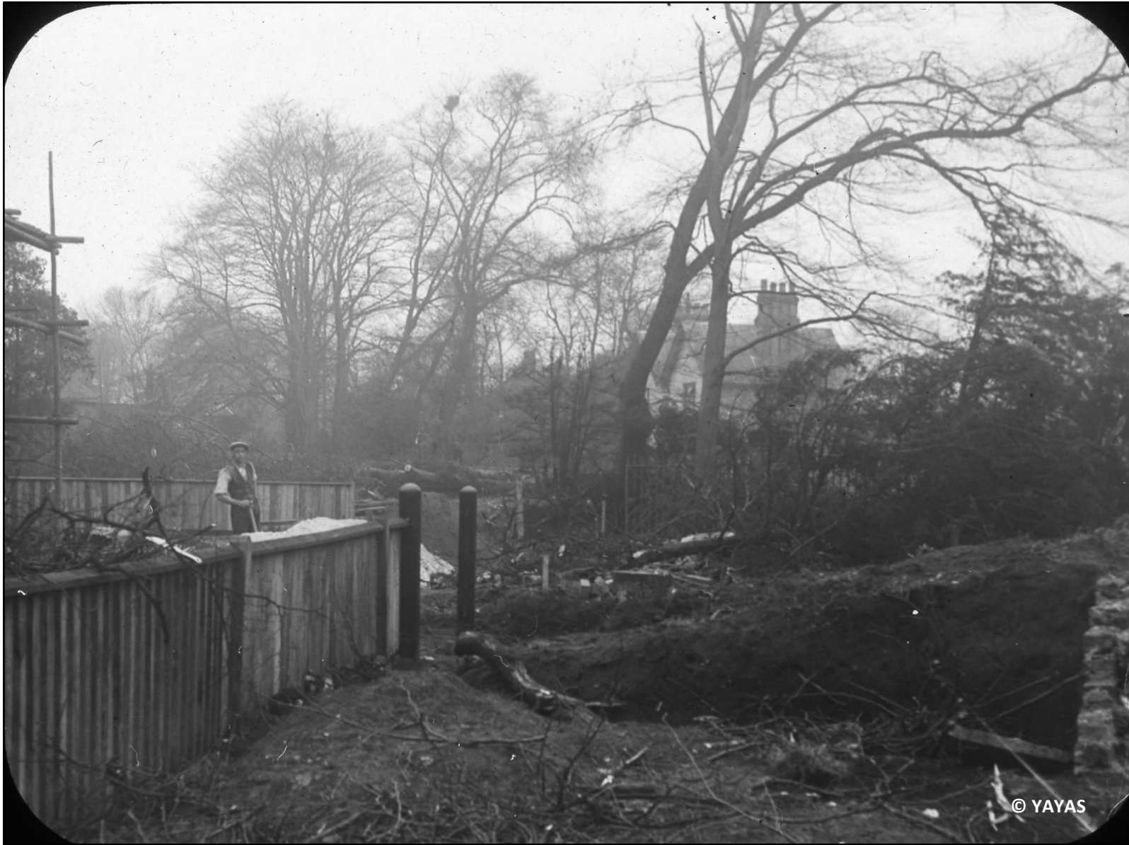
Figure 76. Land clearing and construction on the former Clifton Croft complex, likely 1931-1932. No. 28 Water End, The Sycamore Cottage (now the White House), can be seen on the right-hand side of the photograph, with the Laborers' Cottage behind the figure standing (YAYAS EV2756).
