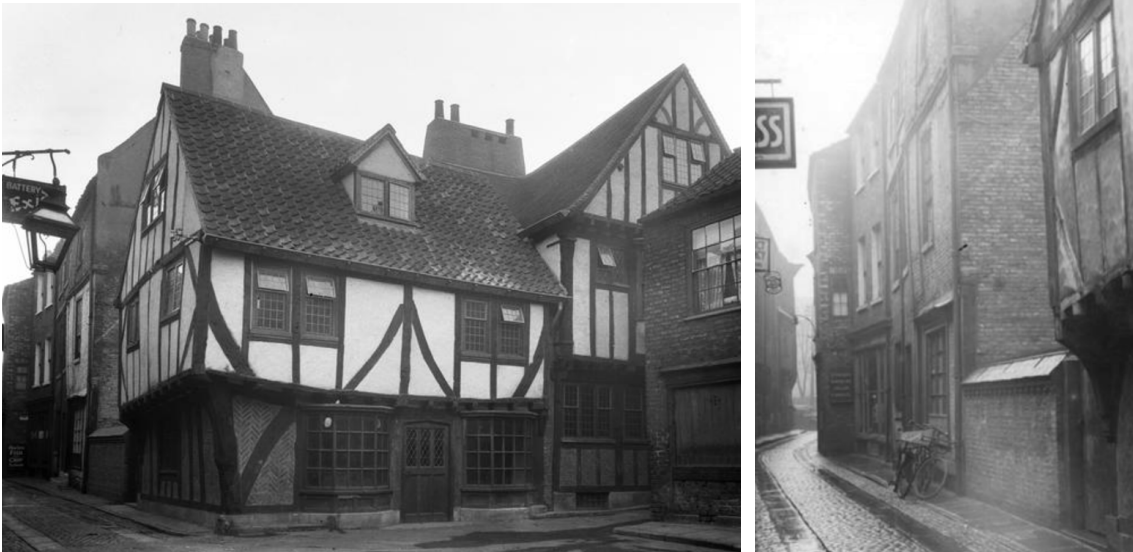
Fig. 4.14 Left - the site shortly after its restoration by Brierley and Rutherford architects for Cuthbert Morrell. Note the creation of a yard on Newgate (left), and in the foreground, the C18th ranges on the south side of Jubbergate have not yet been cleared; Right - detail from a 1933 photograph showing the roof scar of the now lost brick range on the site of the present kitchens © York Explore
