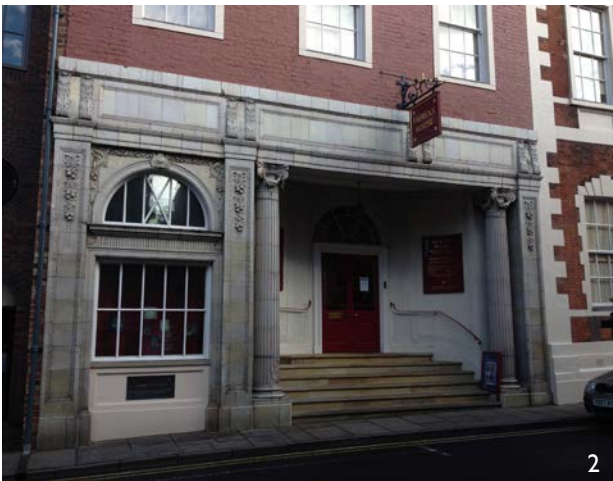
1 The front elevation of Fairfax House on Castlegate (courtesy of Fairfax House)
