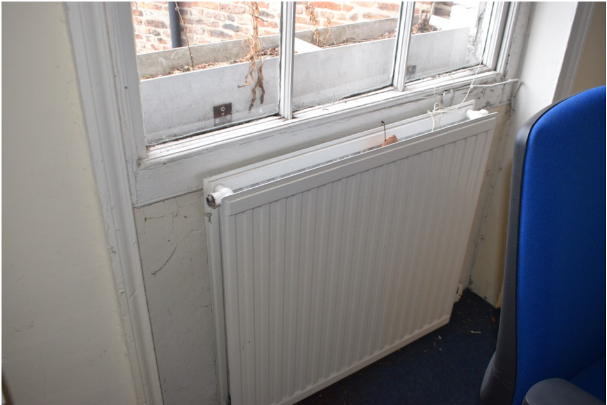
Figure 117: 2 nd floor front room window architraves that extend to the ground (Author 2022).
