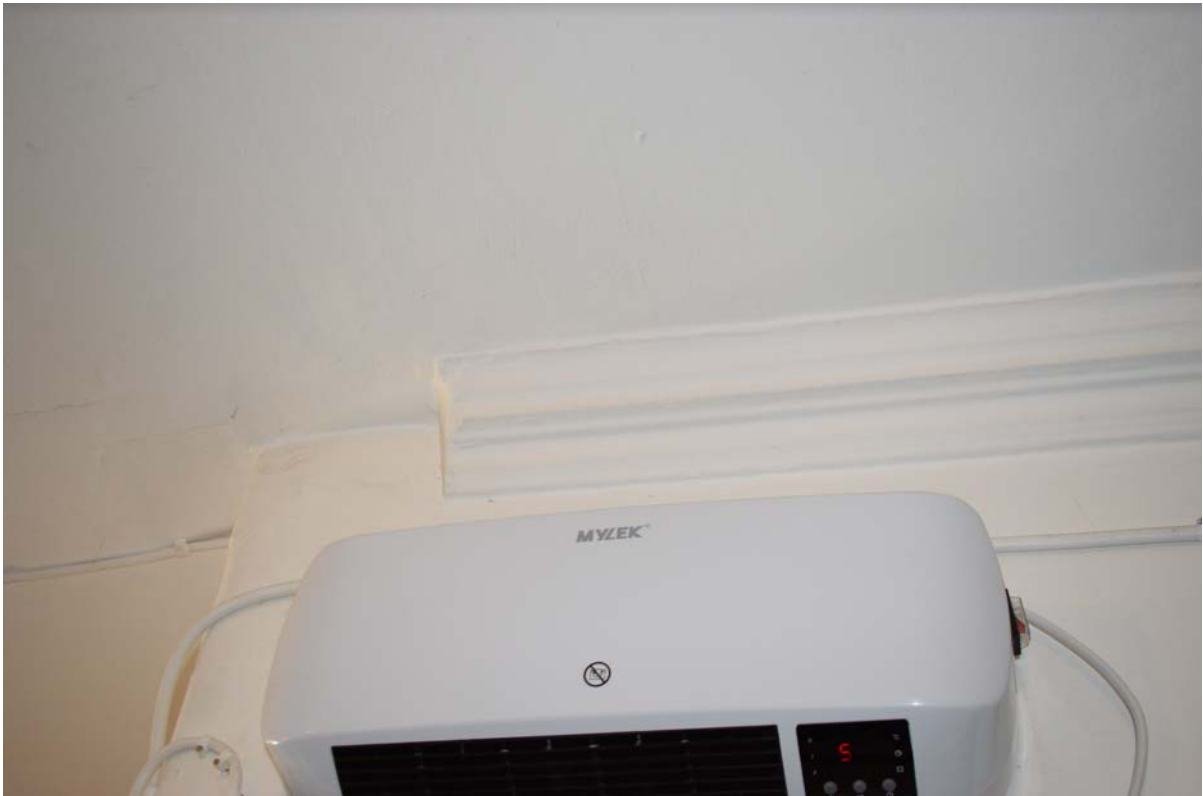
Figure 20: Remains of cornice in drawing room near doorway (Author 2022).
