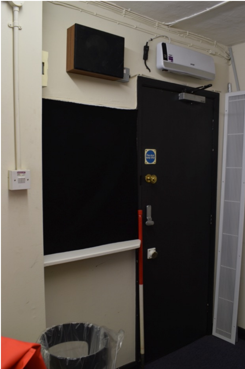
Figure 73: Current doorway into front room. This entrance way has been created in the 20 th century. This area would have been a part of the kitchen in the 18 th century (Author 2022).
