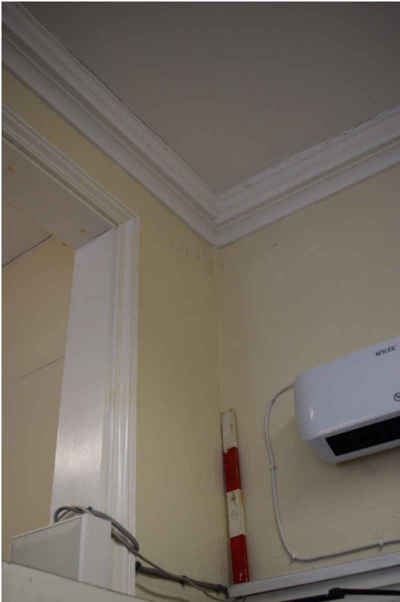
Figure 118: 2 nd floor front room cornice detail in north-west corner (Author 2022).
