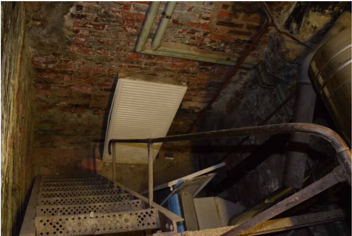
Figure 65: Cellar looking south (Author 2022).
