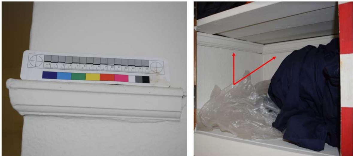
Figure 9: Picture rail runs the full length of the room and is located within the cupboard (Author 2022).
