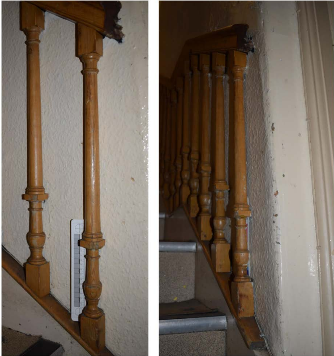
Figure 15: Staircase from ground floor to 1 st floor. The balustrade has been cut off when the entrance was altered in 1901 (Author 2022).
