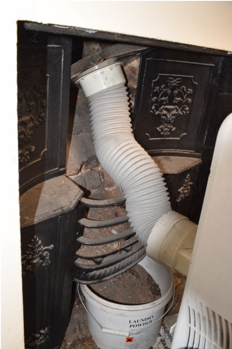
Figure 92: 18 th century fireplace in situ in 1 st floor rear room (Author 2022).
