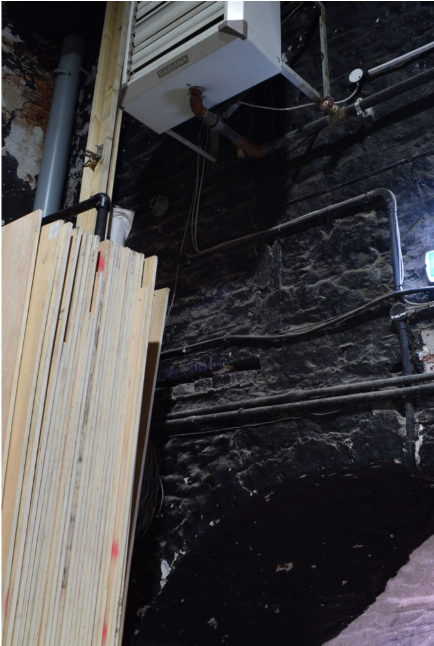
Figure 60: Looking south, blocked up 1 st floor doorway (Author 2022).
