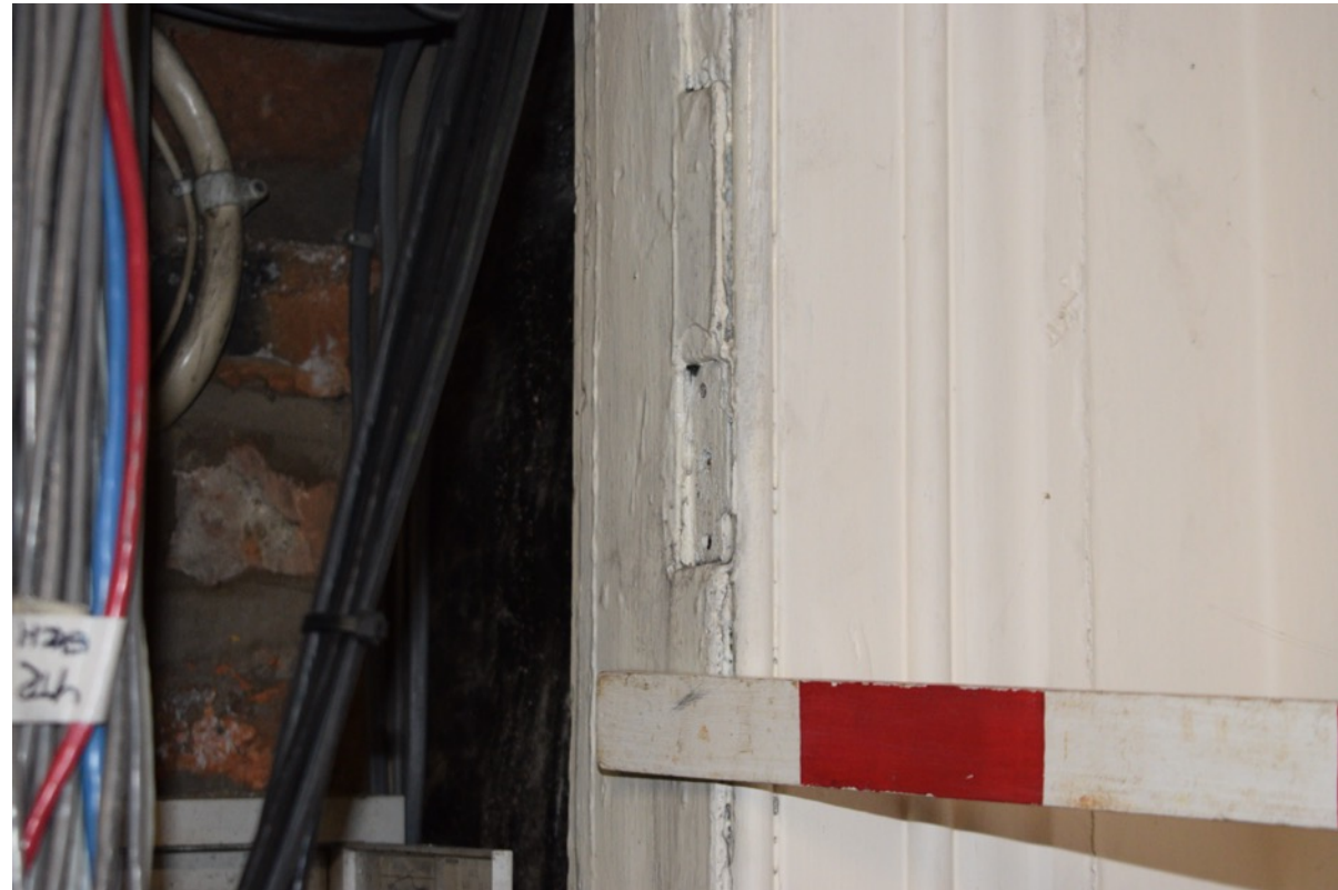
Figure 91: North-east facing corner of 1 st floor rear room (left). The blocked-up doorway would have provided access to a suite of rooms that lay to the north. These northern rooms have been demolished. Detail of doorcase (right) (Author 2022).
