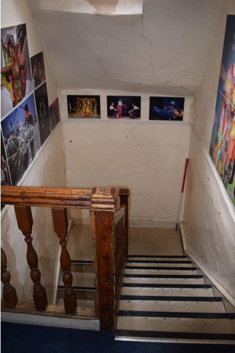
Figure 100: 2 nd floor staircase looking east (Author 2022).
