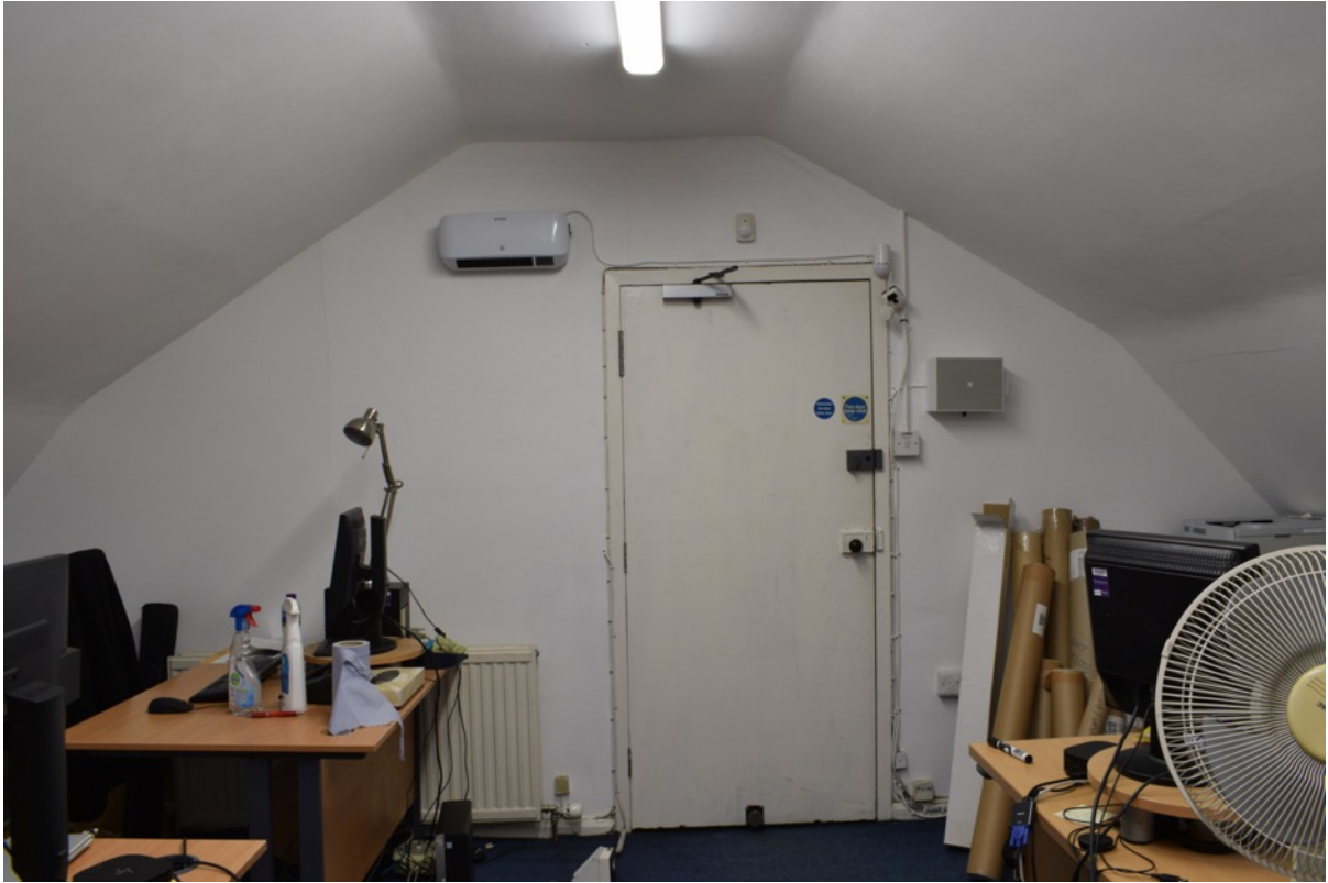
Figure 106: 2 nd floor rear room looking south (Author 2022).
