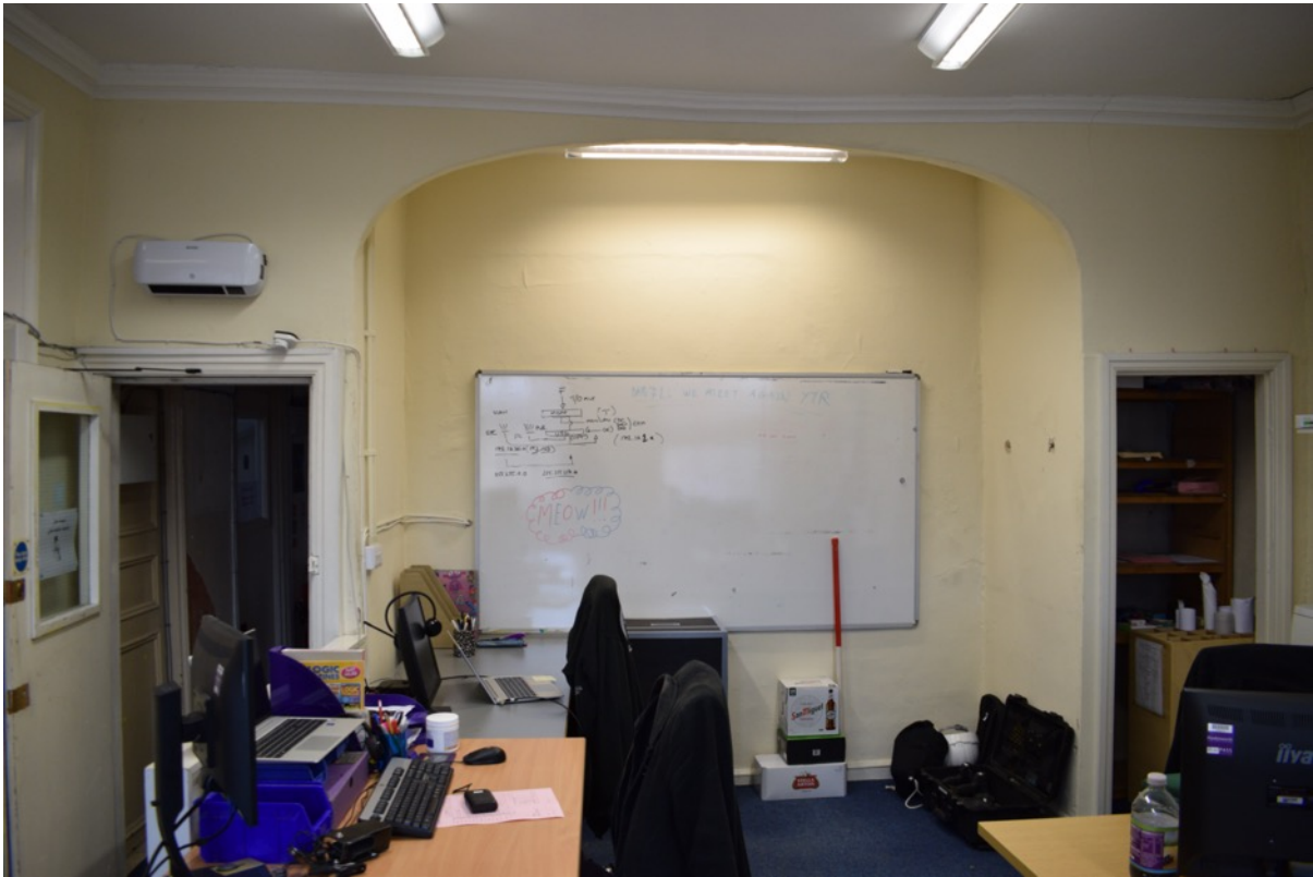
Figure 115: 2 nd floor front room looking north showing bed niche (Author 2022).
