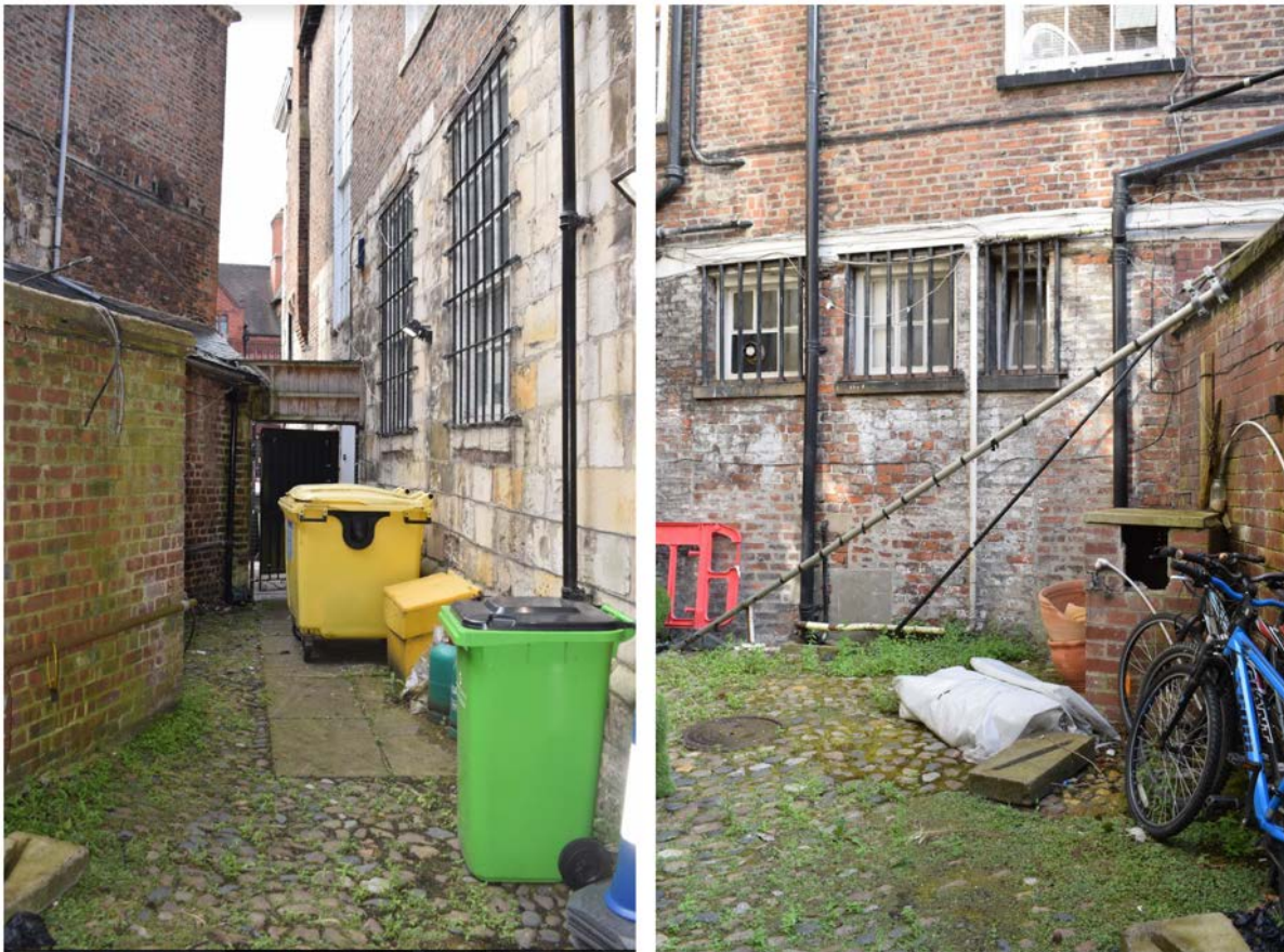
Figure 13: Yard bounded by the TWH, Red House and TRY. Left: Looking south-east towards Duncombe Place, small brick building is a 20 th century addition. Right: Looking north at the external wall of the TRY. The TWH is located to the east. The ground floor immediately in front was not present in the 18 th century with the 1 st floor constructed on piles (Author 2022).
