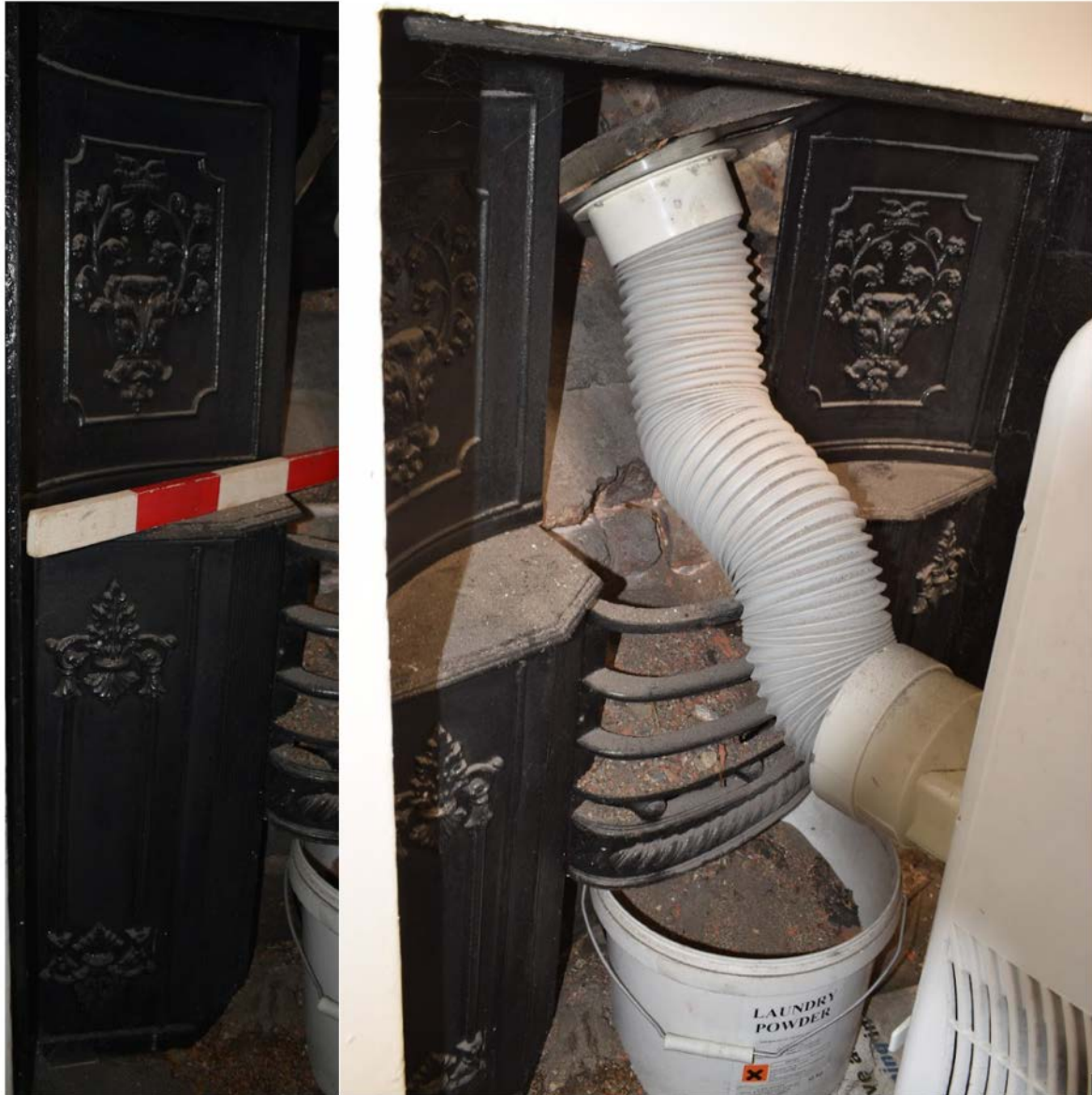
Figure 23: Fireplace in south-east corner of the dining room with decorative iron hob grate in situ (Author 2022).
