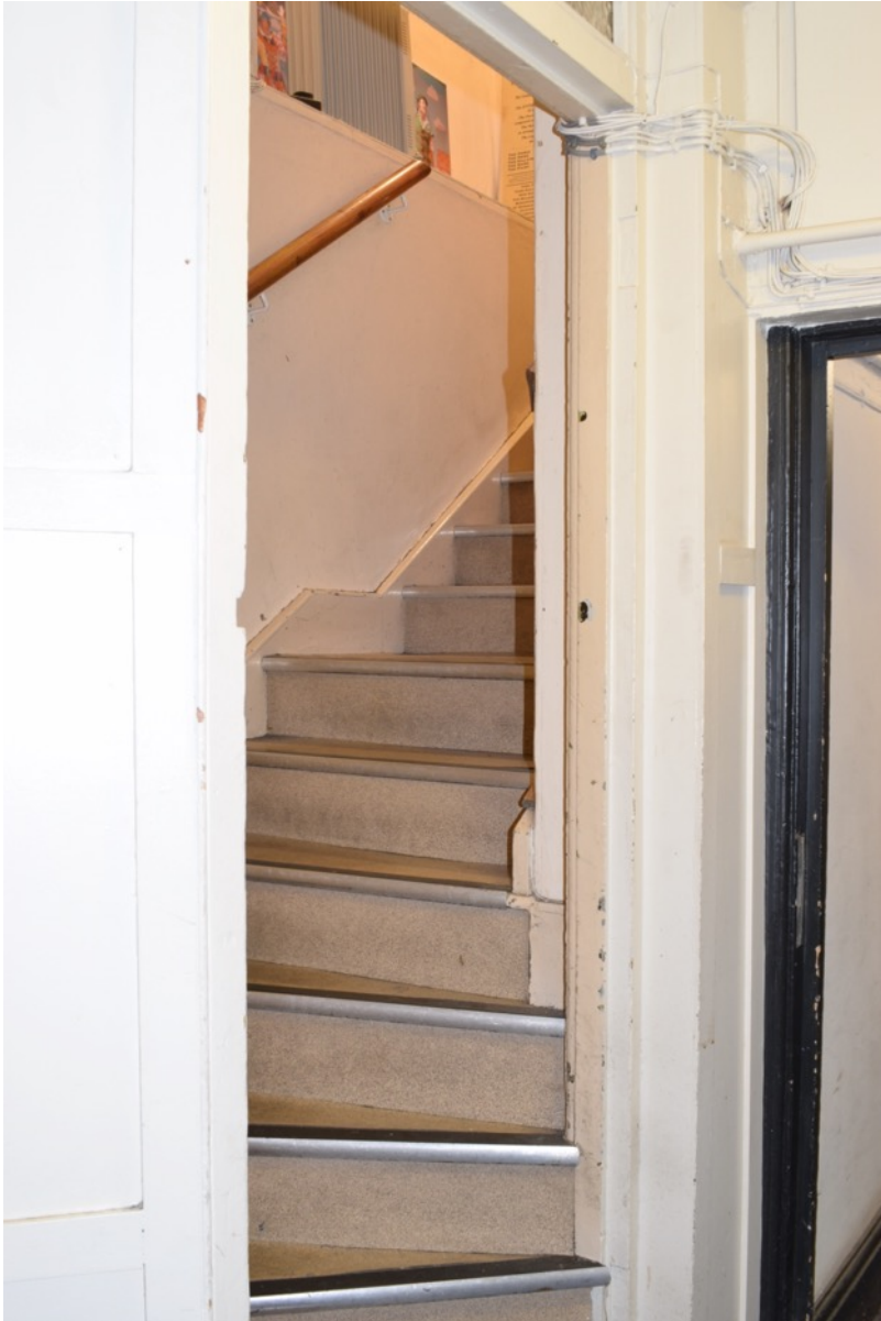
Figure 76: Base of staircase to 1 st floor in entrance lobby of the TWH along west wall (Author 2022).
