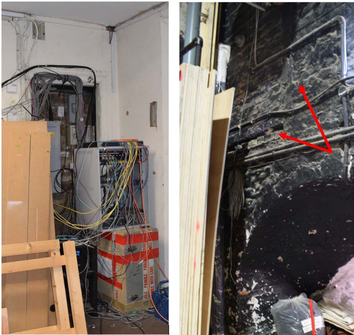
Figure 24: Blocked up doorway that would have led to the guest bedroom. The interior door is difficult to access due to equipment in the room. Remains of the door can also be seen from within the room that was the scullery on the ground floor (Author 2022).
