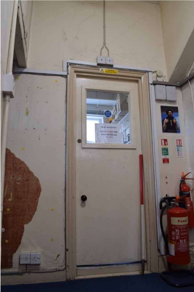
Figure 102: 2 nd floor landing looking west. Door to western side room (Author 2022).
