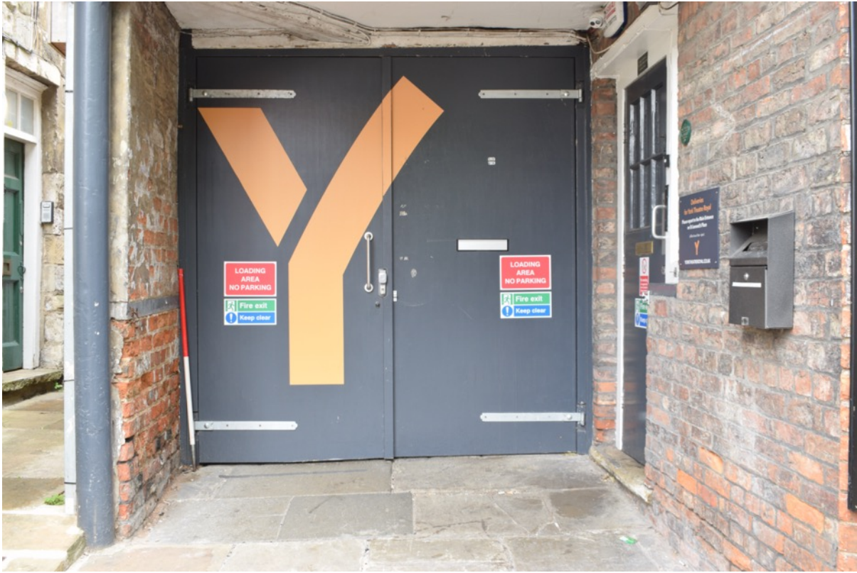
Figure 119: Exterior entrance to get-in on southern elevation (Author 2022).
