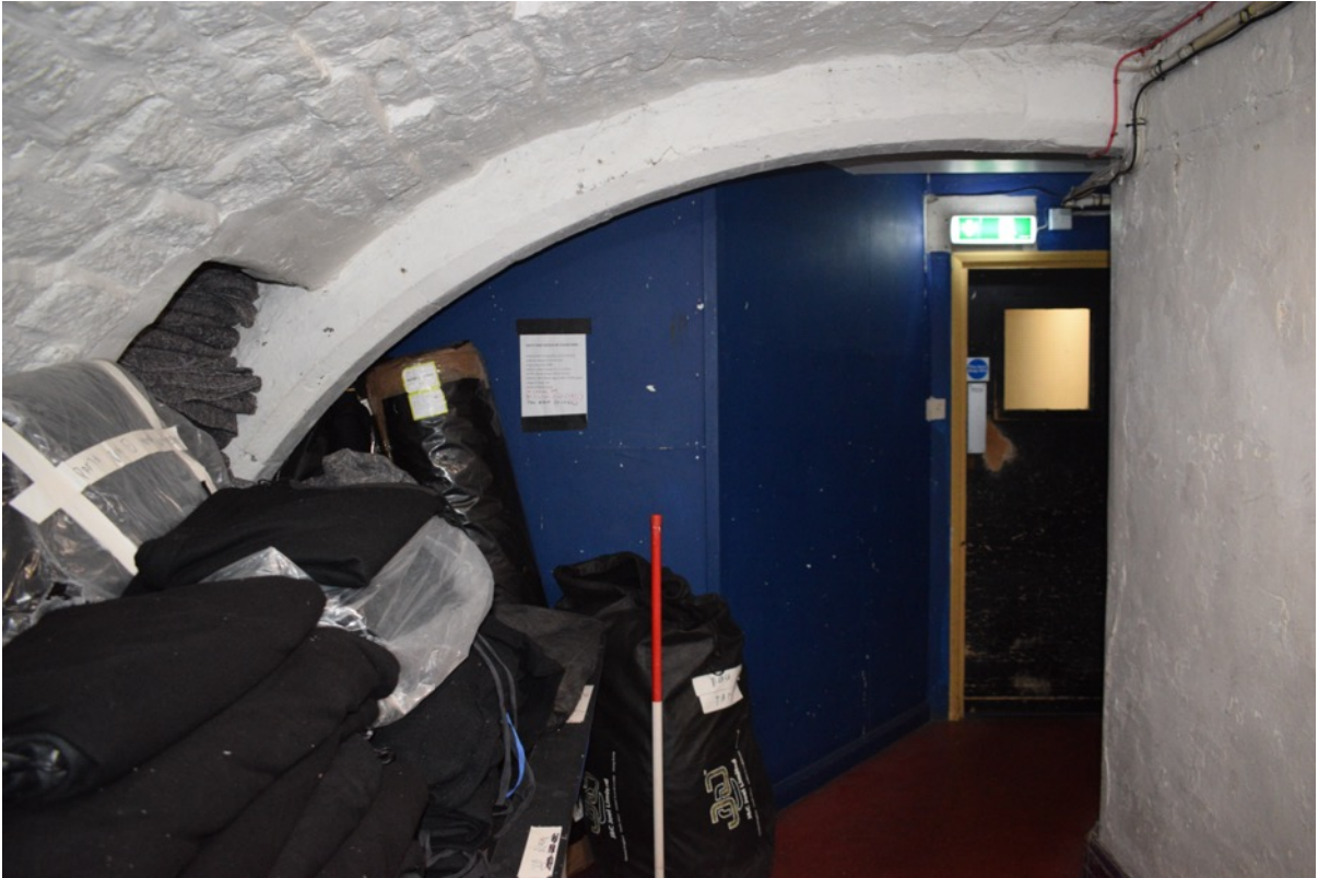
Figure 63: Location of 18 th century scullery, looking south (Author 2022).
