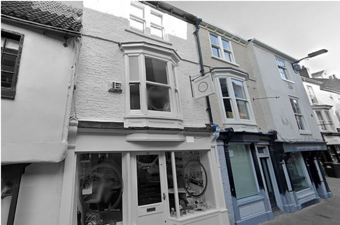
Fig. 5.2 Two main front elevations of no. 60 Goodramgate to right, with no.62 and Lady Row to the left.
