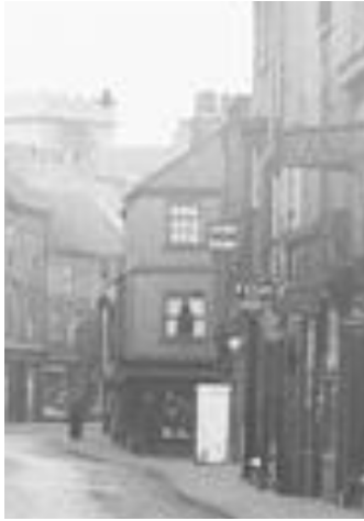
Fig. x Detail from a 1930s photo, showing the return elevation of the site, with curtains in the upper windows, and seemingly decorated in a darker paint colour than today including distinctive sill bands (© York City Archives).
