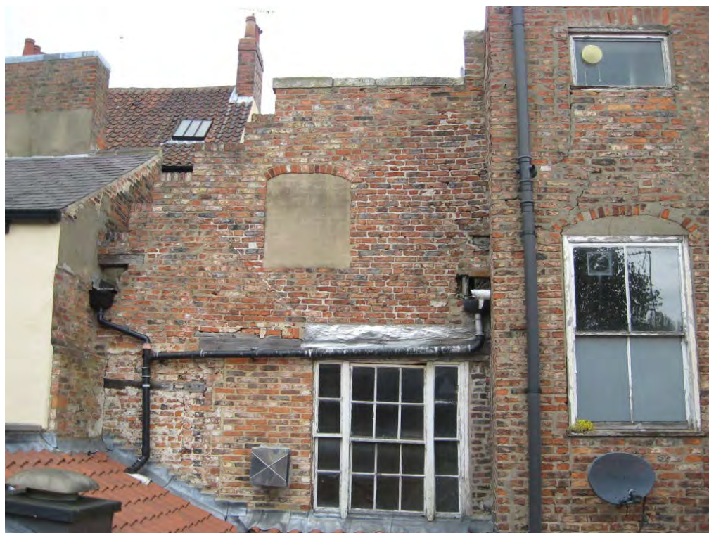
Plate 4. The west side of the rear elevation
